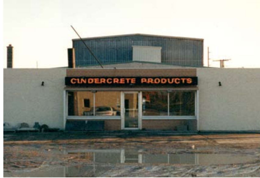
A modern Cindercrete plant opened in 1964 on Highway #1 just east of Regina.
