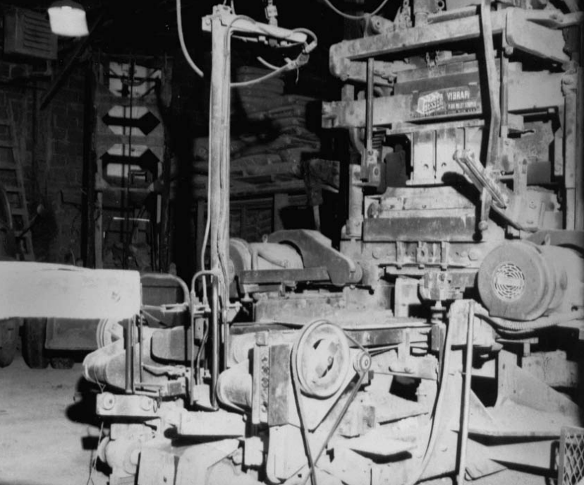
Besser block machine that advanced mechanization at Cindercrete in 1951.
